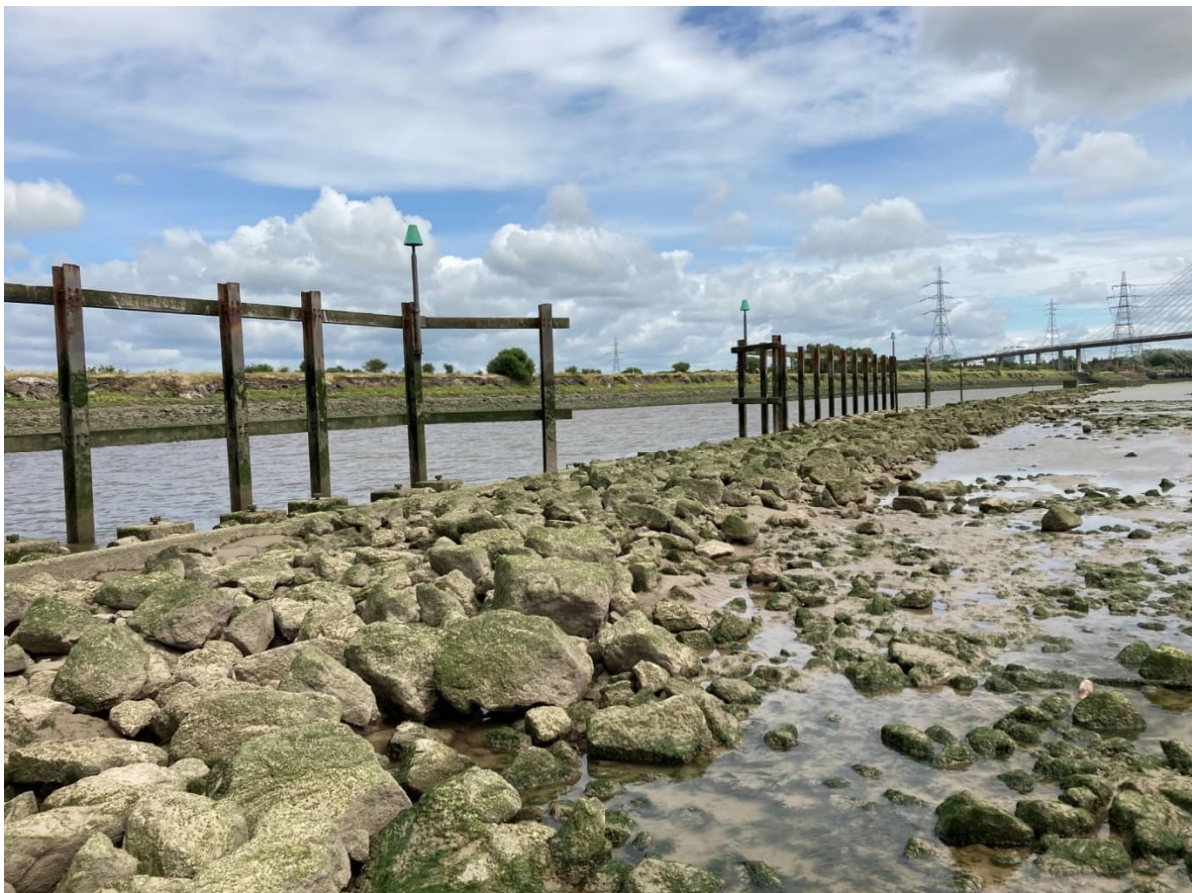
Plate A-13: Boulders placed around outfall infrastructure
